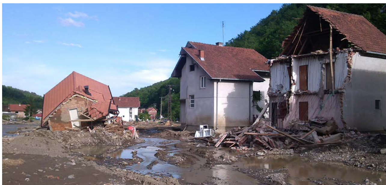
Figure 3.2 Flood and mudslide damage to houses in the town of Krupanj, Serbia, 2014
